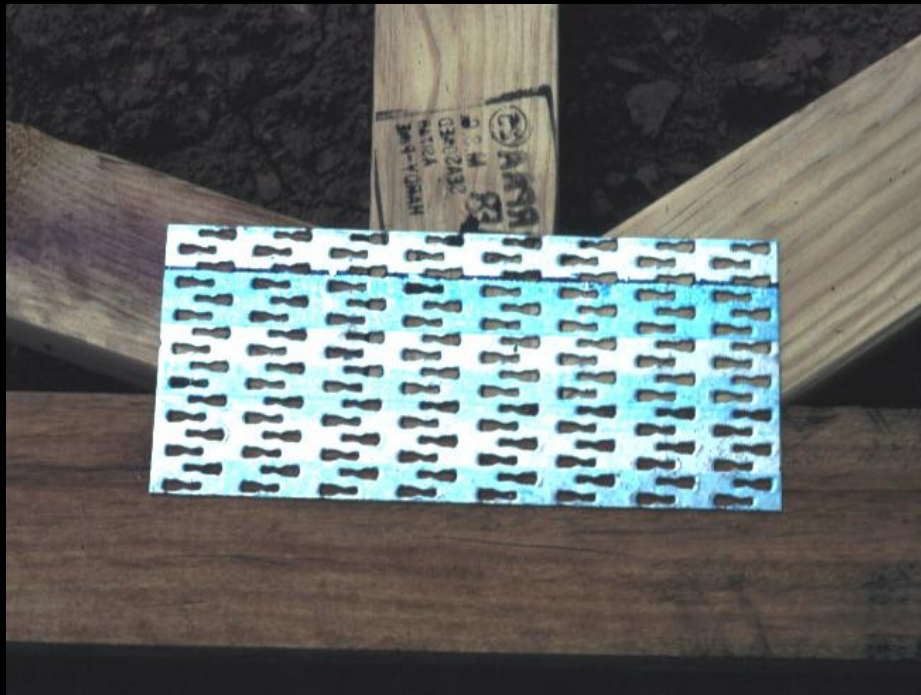
Nailplate joint
