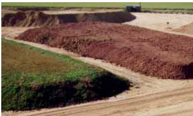
Clearly defined stockpiling of different soil materials
