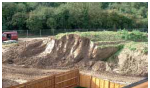
Long term stockpile of stripped topsoil left with only weed vegetation
