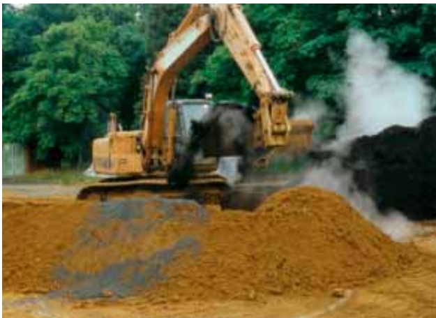
Blending organic matter with mineral material
