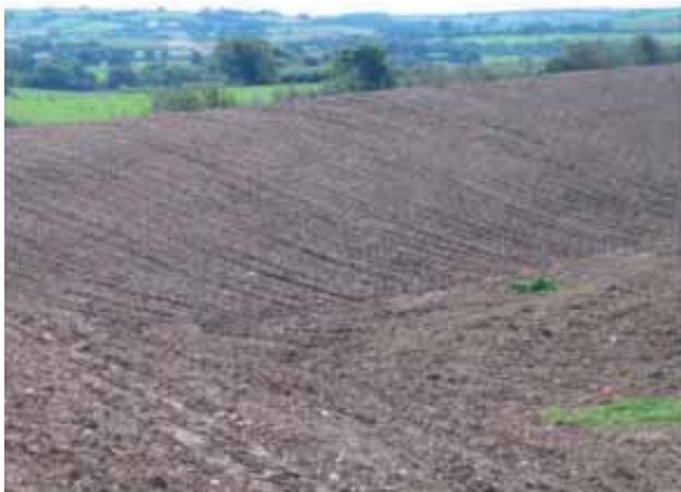
Permanent storage created for surplus topsoil stripped from a greenfield site in Devon, despite there being demand for topsoil in the locality.
