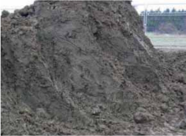
Topsoil stockpiled when wet and plastic
